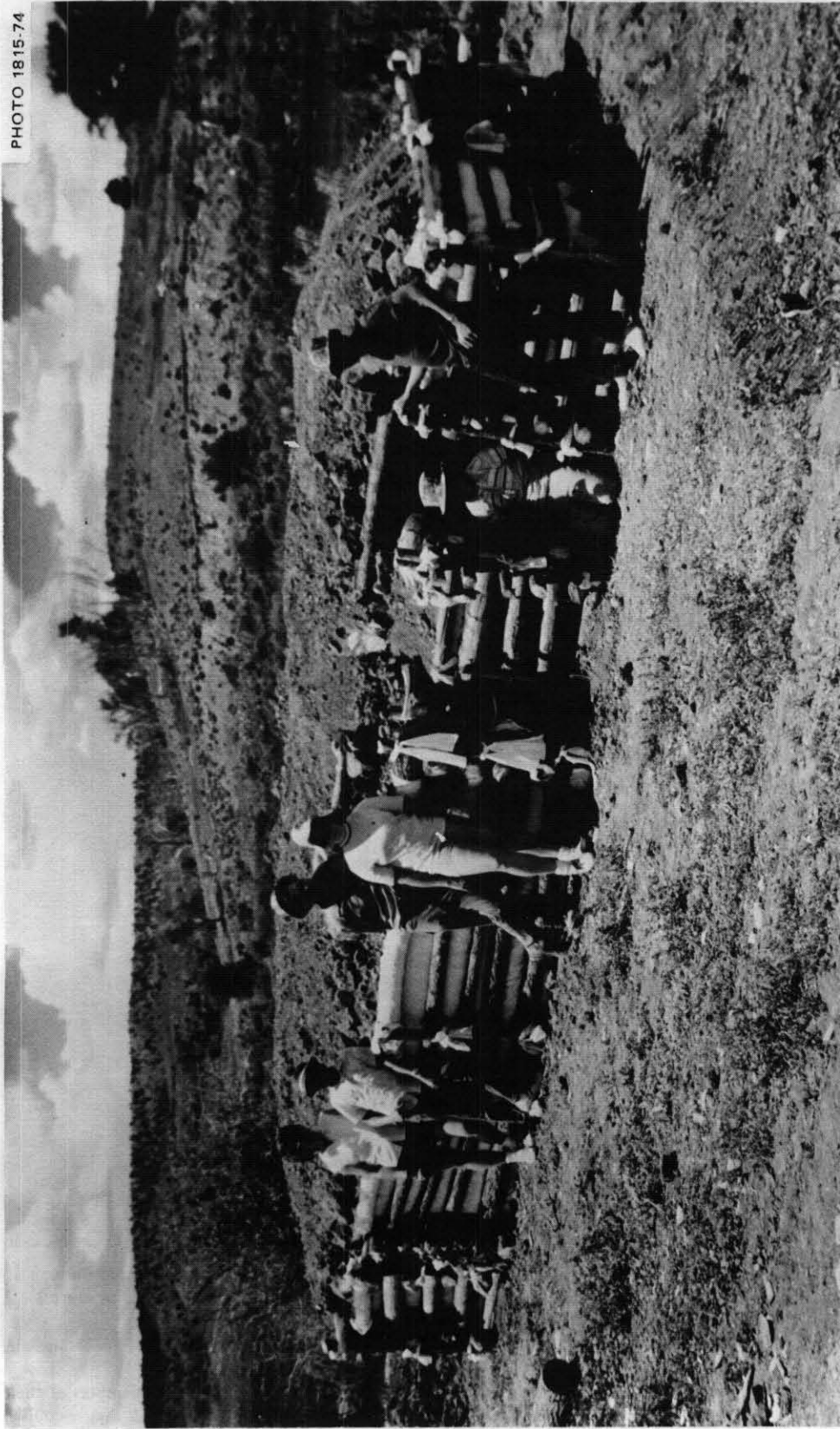
Fig. 5.27. A Crib-Walled Shelter completed in Colorado. This family finished 29 hours and 53 minutes after receiving the building instructions at their suburban-type home about 9 miles away from this site. All six members were at this site, working over 90% of the time, for 10 hours and 13 minutes on May 26th, and for 5 hours and 11 minutes on May 27th. If they had built near a woods and had cut all the poles specified for this shelter, Kearny believes this family could have finished it by working as hard for two full days, 10 or 12 hours each day.
